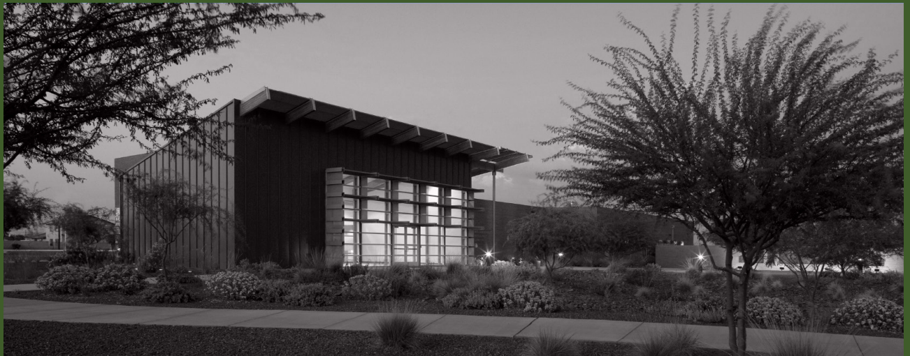
City of Phoenix Neighborhood Resource Center & Police Substation
